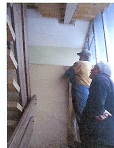
Hmm – large cabinet stuck between floors, before being disassembled
