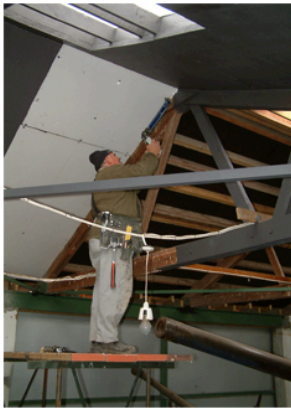
Peter Bulman fitting insulation to the Quartermaster's Store.
